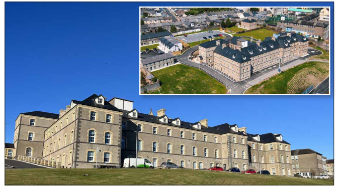
The largest RLS project to date in Waterford is at St Joseph's House on Manor Hill, where 71 homes have been created in a previously vacant convent in a city centre location.
