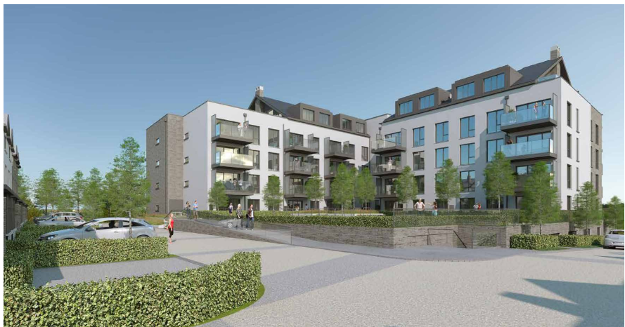
Park Developments' apartments in Dublin – one of the recipients of Croí Cónaithe funding.
